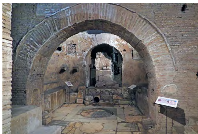
The sanctum where members had been standing shows a floor made with masonry, marble and tiles in a jumbled surface of make do and old bits. Unusual in the grander context of Rome and its glorious marble clad buildings
